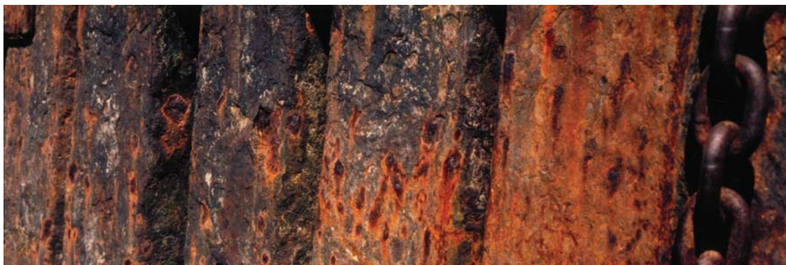
The Columbuskaje before service works in 1985 – extremely corroded
